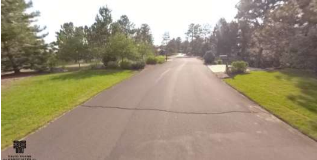
Transverse Cracking
